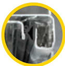
Integrated rain gutter (IRG) construction
