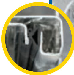
Integrated Rain Gutter (IRG) construction
