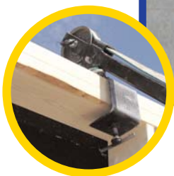
Quick lifting bracket installation
